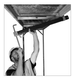
The console clip is installed from underneath the console plate and locks during load.
