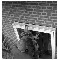
The window is lifted and pushed into place.
