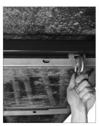
The Upclimber is hooked up to the console clip hoist via carbin.
